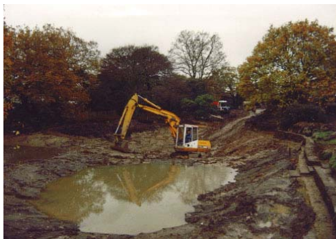
Pond being de-silted during restoration
